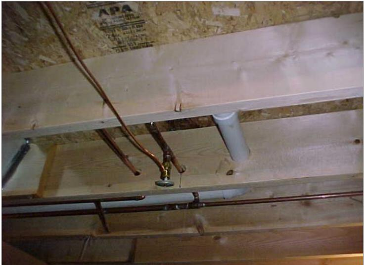
\* Cutting, drilling and notching R502.8
