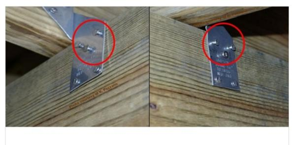
Average withdrawal strength of smooth-shank SS nails is 20% to 50% lower than smoothshank carbon steel nails.
